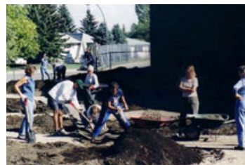
Preparing the ground.
